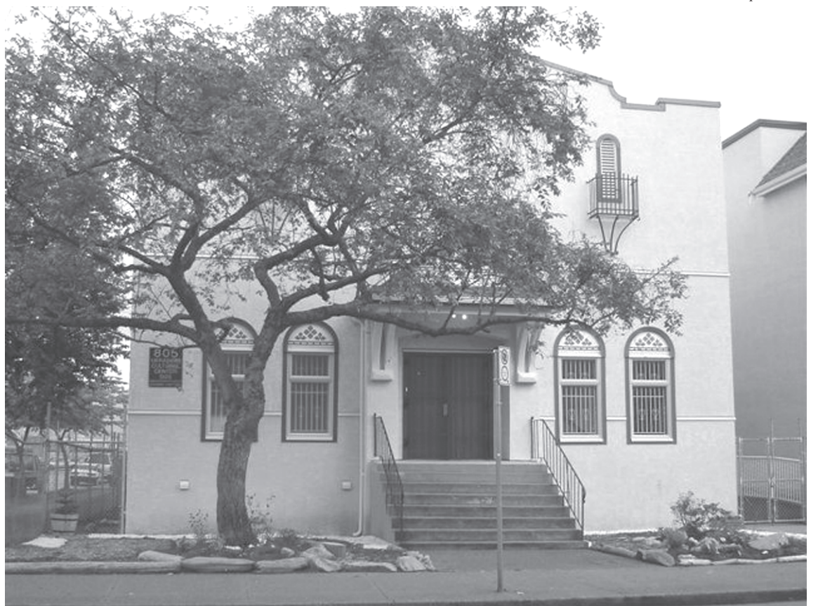
This is the new look of the Ukrainian Cultural Centre at 805 East Pender in Vancouver, with the scaffolding, protective materials and other construction details removed. The interior of the building also had extensive work done.
